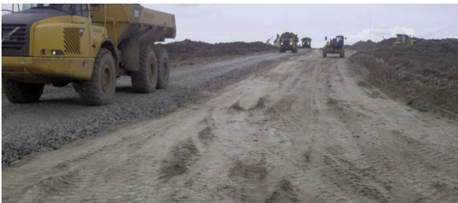
Haul road constructed with Mirafi® HP570 as designed.
