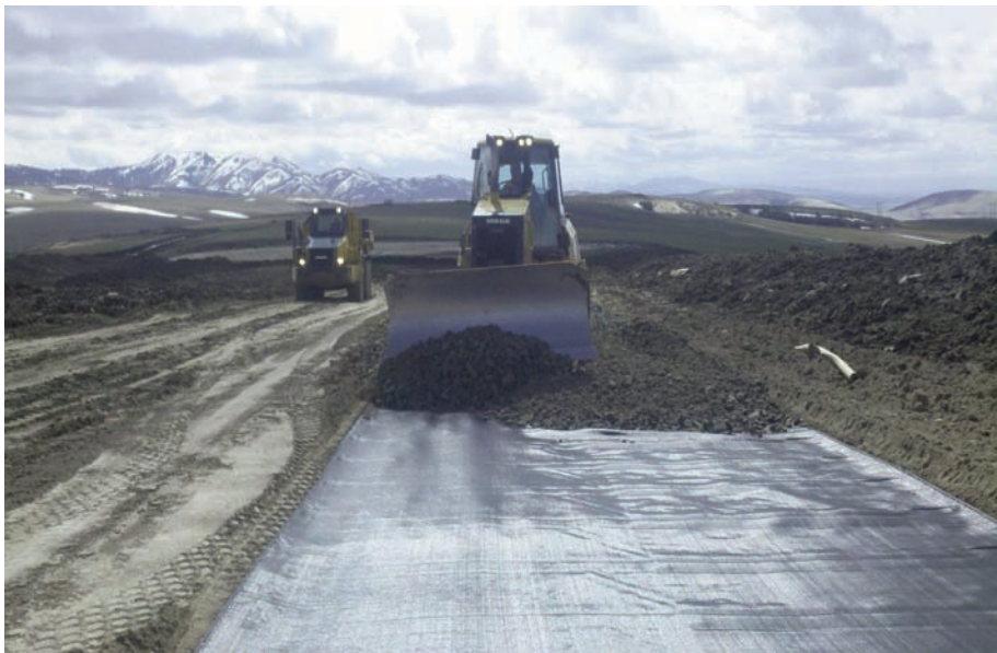
Placement of Mirafi® HP570 and 10" to 12" of 3" minus basalt stone.
