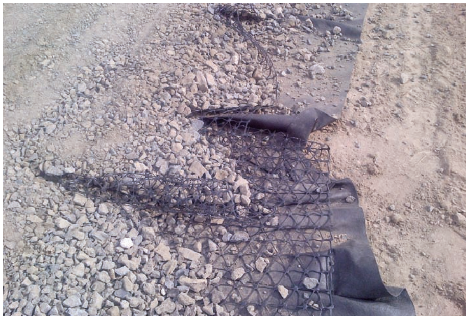
Layer of 4 oz nonwoven and multi-axial geogrid with placement of stone. This picture shows 2 different widths of material with kinks and folds in the material. There is not full geosynthetic coverage over the subgrade surface.
