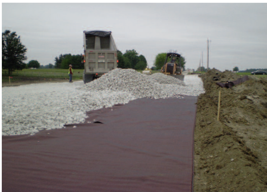
Placement of the 3-inch minus aggregate on Mirafi® RS580i.
