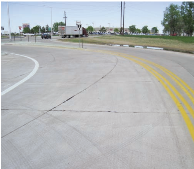
Completed installation of finished pavement on Mirafi® RS580i.
