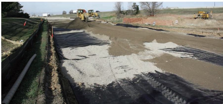
Placement of base material on Mirafi® RS580i.
