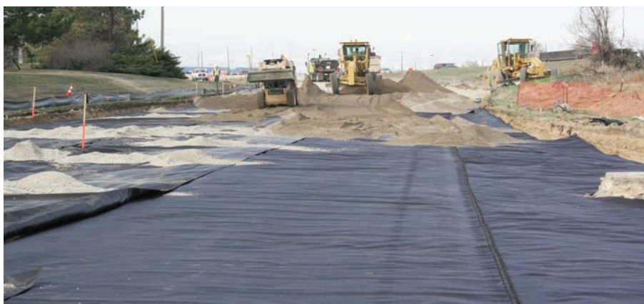
Installation of Mirafi® RS580i.
