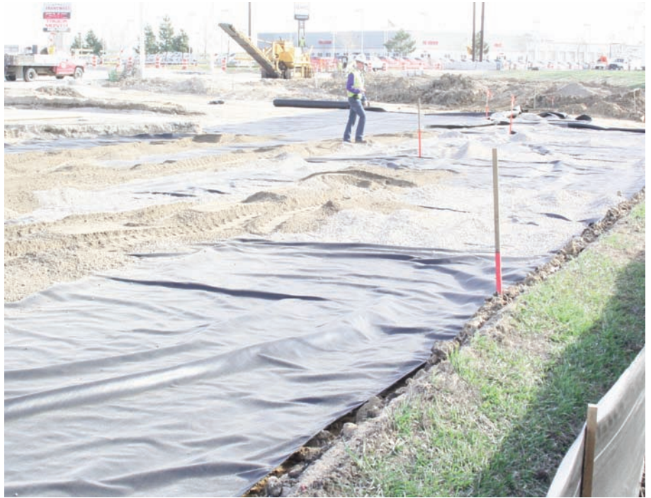
Placement of Mirafi® RS580i looking East .
