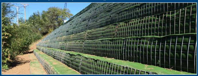
Cherry Island Landfill is one of the largest vertical expansion berms in North America, measuring over 65' tall and almost a mile long. The reinforced berm utilizes high-strength geotextile material with a tensile strength of over 80,000 lb/ft.
