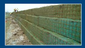
TenCate Miramesh® geogrids provide some of the highest UV durability reinforcement available, allowing for permanent green face walls and slopes.
