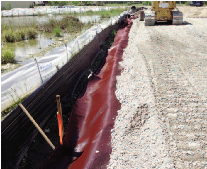
Leveling the compacted lift of Limerock Base aggregate on Mirafi® RS580i before placing Mirafi® BXG12. Finished flexible pavement surface.
