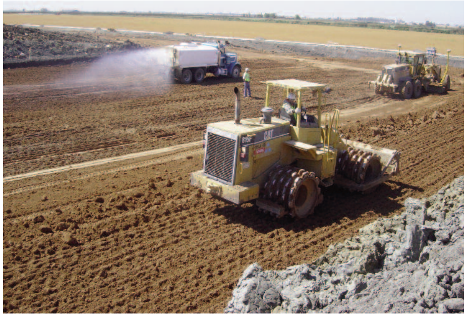
Soil was placed and compacted over each layer of geogrid.
