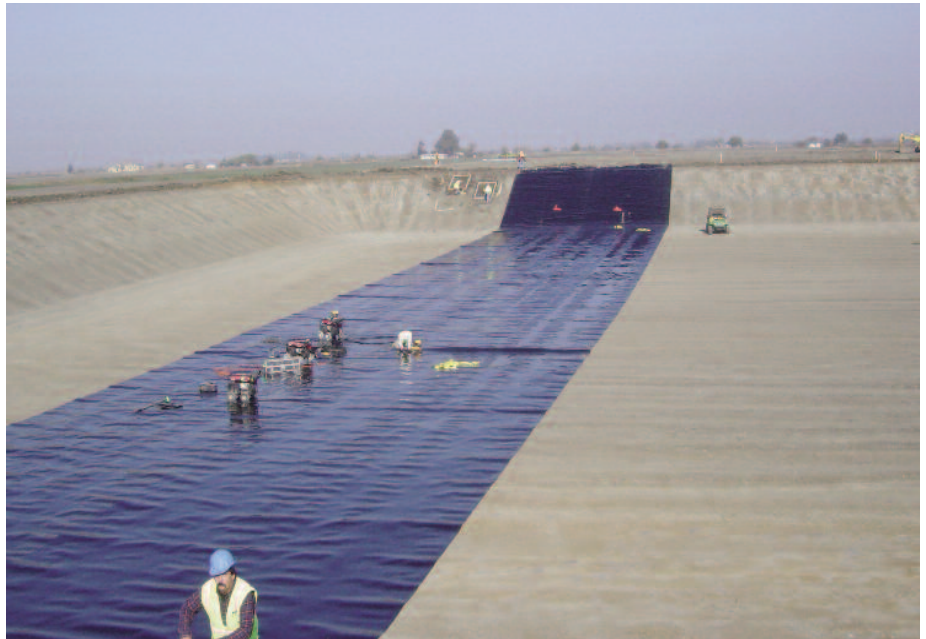
Finally, an impermeable liner was installed to complete the pond installation.
