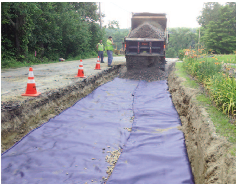
Placing 12" layer of 1 1/2" < stone.
