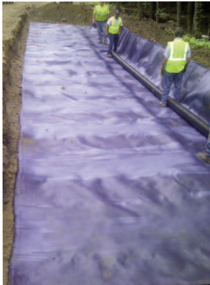
Mirafi® H 2 Ri geosynthetic undergoing installation.
