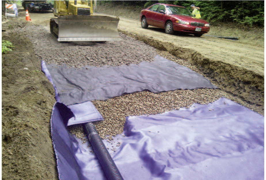
Placing lift of 3" < over Mirafi® 160N.
