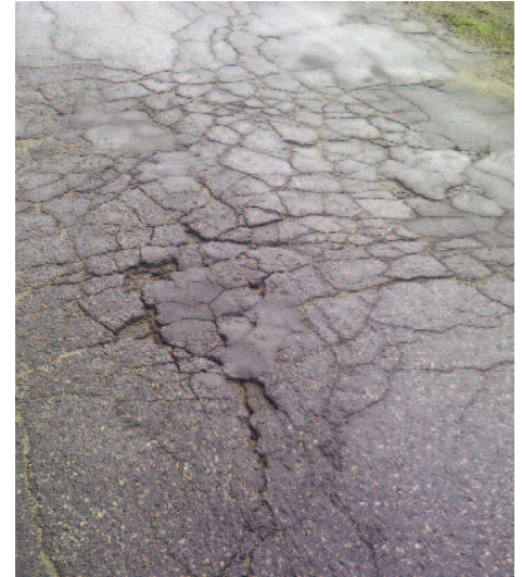
Condition of roadway prior to construction.
