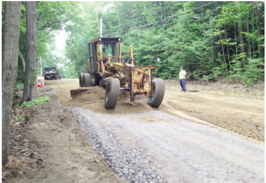
First layer of 1 1/2 < before pavement overlay.
