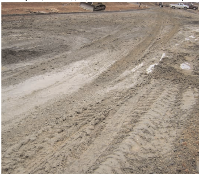
Subgrade conditions prior to the placement of Mirafi® HP570.
