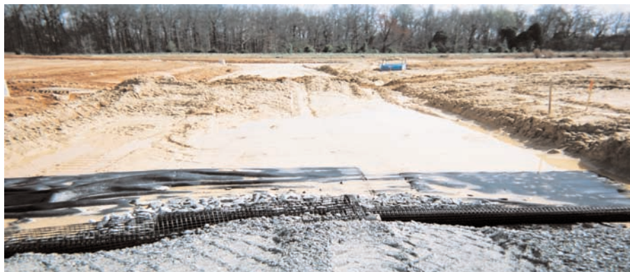
East Road subgrade conditions prior to placement of geotextiles.
