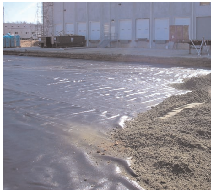
Starting placement of Mirafi® HP570 and base course under asphalt pavement adjacent to the concrete truck dock area.
