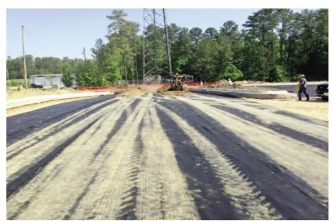
Installation of base course aggregate over Mirafi® HP570 geotextile.
