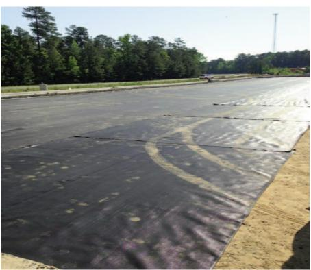
Installation of Mirafi® HP570 geotextile.
