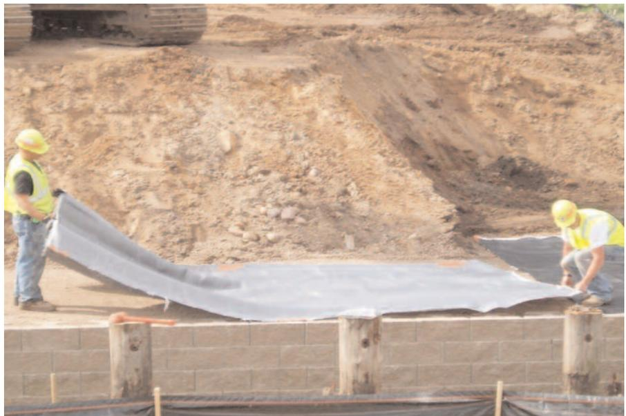
Placing the Mirafi® PET770 reinforcement layer.
