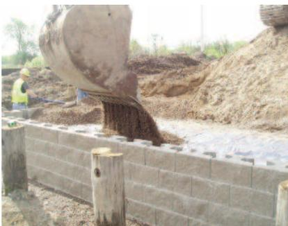
Backfilling behind the precast block. The geotextile, block, and aggregate work together to form a reinforced earth system.
