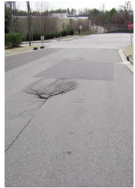
Parkstone 2011: Pavement deterioration continues where the area was replaced.
