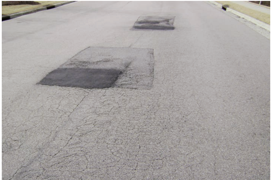
Country Trail without Mirafi® HP370 in 2011 already had areas re-sealed and shows signs of major alligator cracking.
