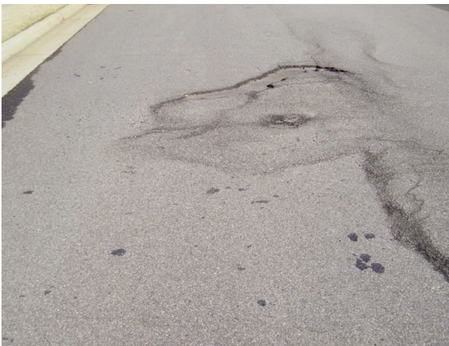
2007: Without the benefit of geosynthetics, Parkstone showed signs of premature deterioration.
