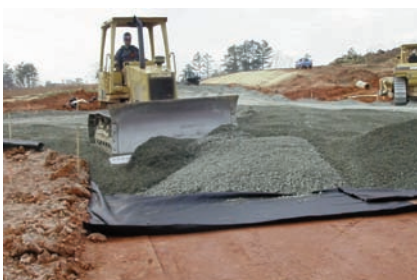
Mirafi® HP370 and base course being placed on the relatively firm subgrade.
