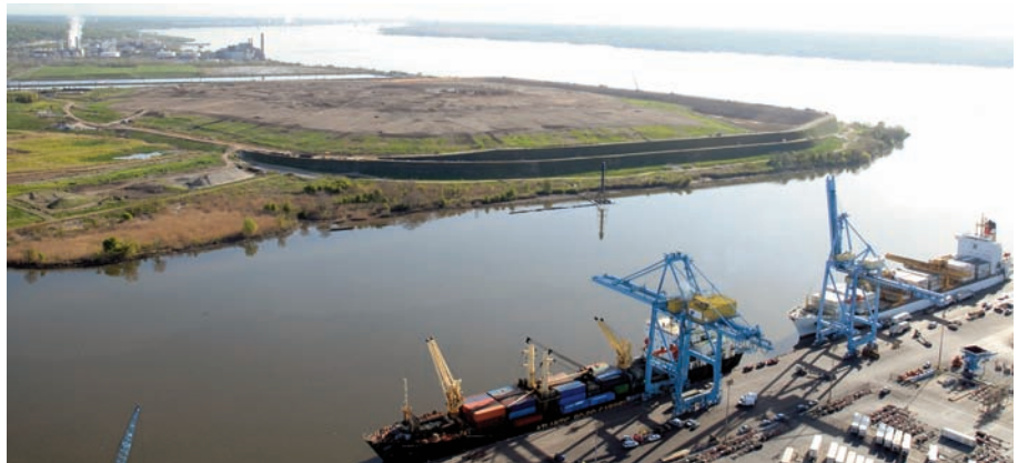
Completed berm looking across the Christina River.
