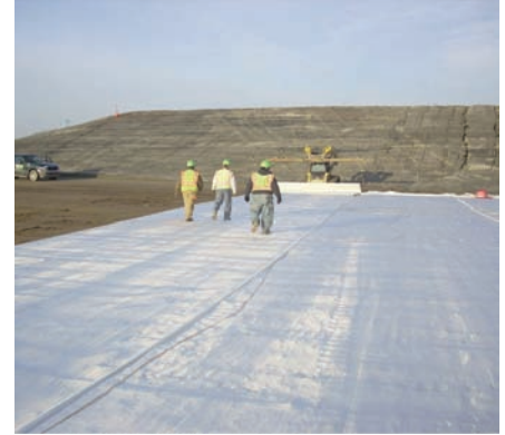
Installation of the first layer of Mirafi® PET1170
