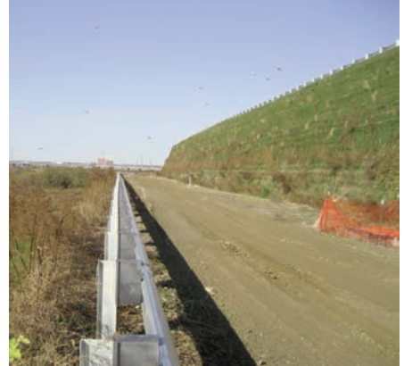
Lower tier of berm and access road, approx. 25% complete.
