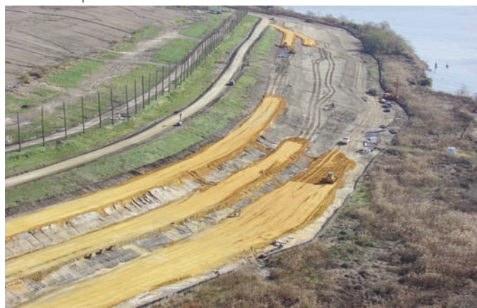
Beginning of berm construction: Installation of PVD's and sand layer.
