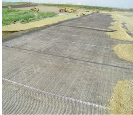
Installation of Miragrid® 20XT.
