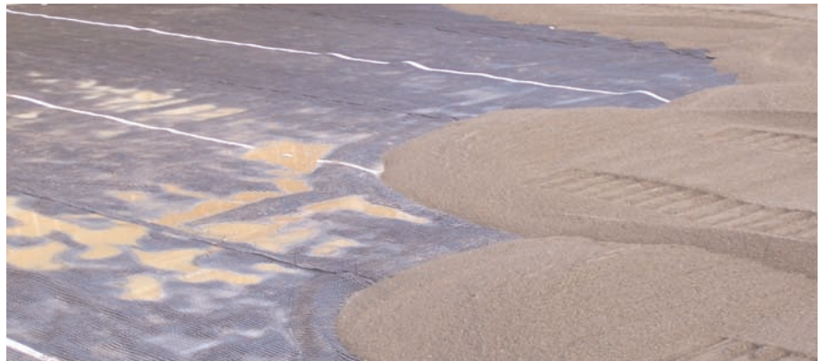
Crushed rock placed directly on Miragrid® 24XT over saturated finegrained soils.
