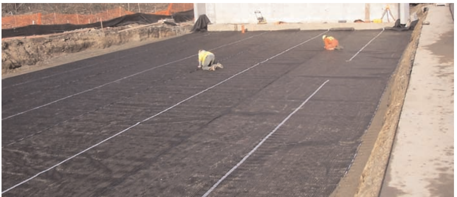
Placement of Miragrid® 24XT with 0.3-meter overlap and zip ties every 1-meter.
