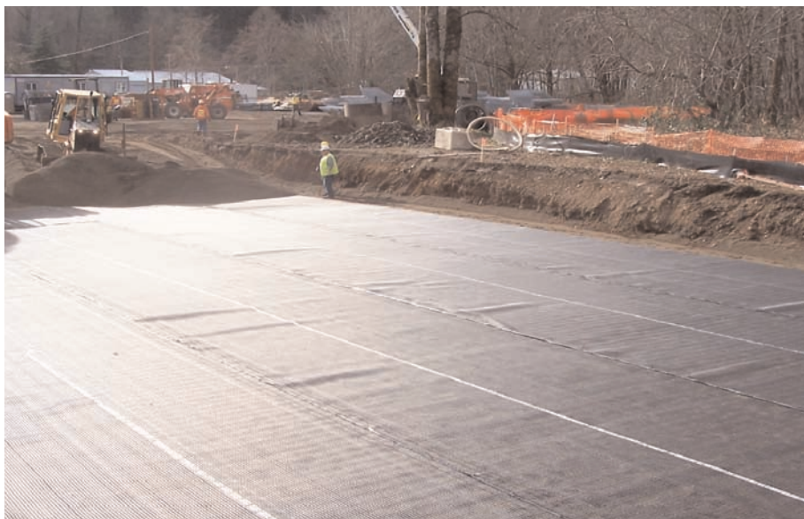
Fourth lift of Miragrid® 24XT, which provided a stable platform for constructing the southern bridge approach.
