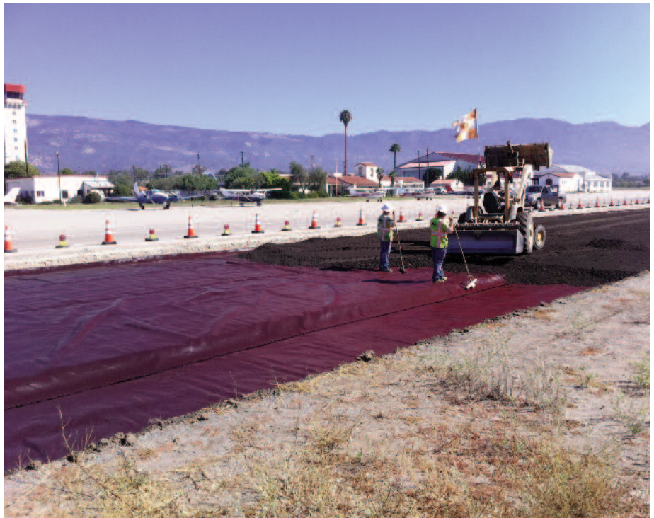
Workers help spread the asphalt grindings evenly over Mirafi® RS380i high strength geotextile.
