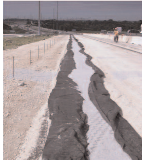
Backfilled drainage trench.
