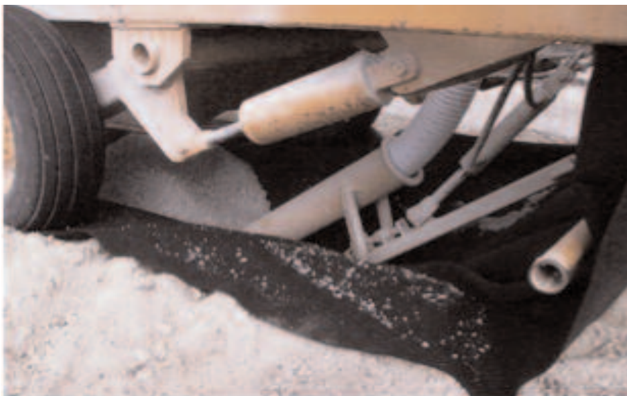
Mirafi® 140NC, Big "O" pipe and drain rock being installed.
