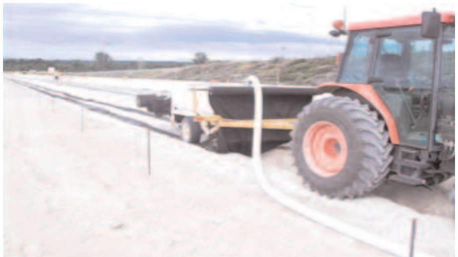
Tractor drawn hopper with Mirafi® 140NC, Big "O" pipe and drain rock.
