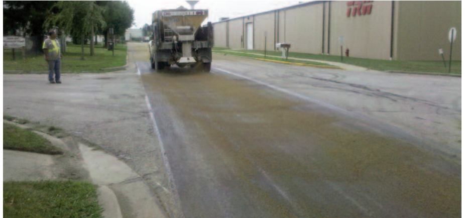
Sanding the Mirafi® MPV500 paving fabric.
