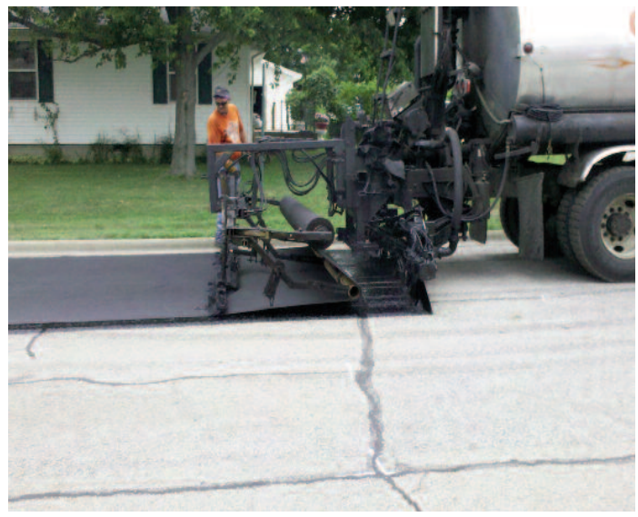
Tack coat and Mirafi® MPV500 being installed.
