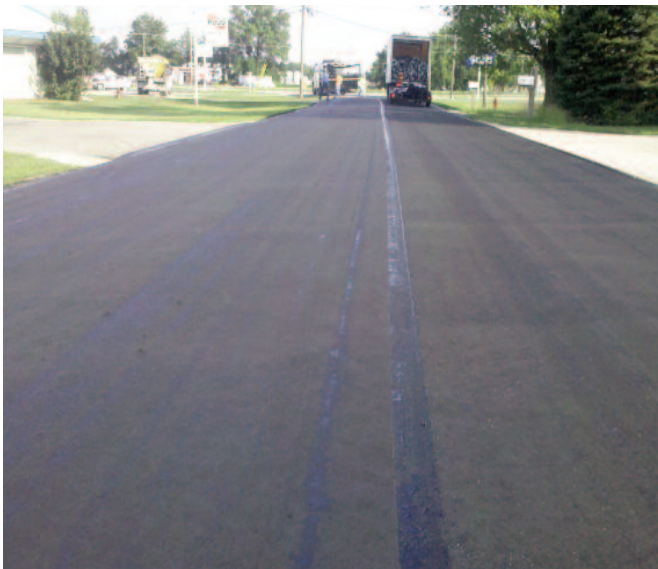
Installation of Mirafi® MPV500.
