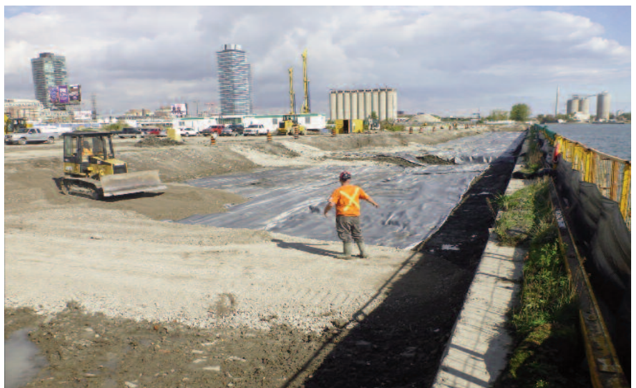
Blading out the aggregate on top of Mirafi® HP770PET.
