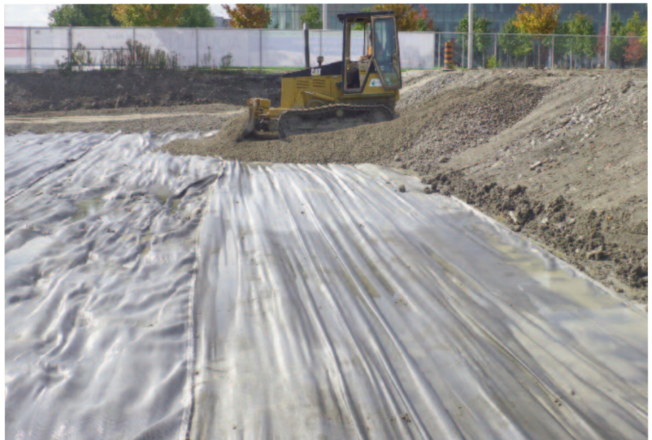
Bridging soft soils and building the platform.
