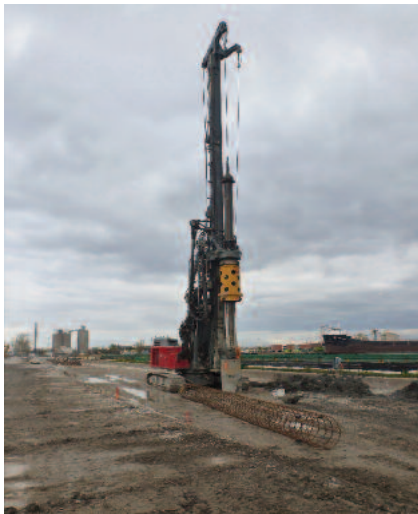
Driving piles on the reinforced platform.
