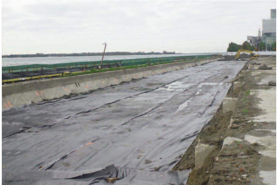
Two feet of overlap was needed when placing the Mirafi® HP770PET.
