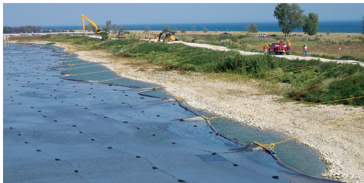
High seam strengths are critical to the field performance of the panels to prevent rupture during fill placement over the low-bearing capacity sludge/ash.
