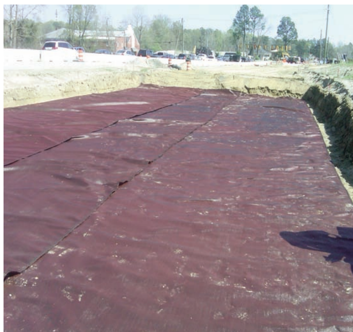
Mirafi® RS580i placed over the soft subgrade areas.
