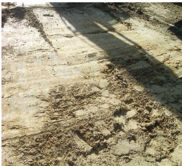
High plasticity clay (CH) subgrade soils after removing previous sandfill.
