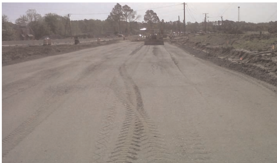
Placement of the base course aggregate over Mirafi® HP270 prior to the proof roll.
