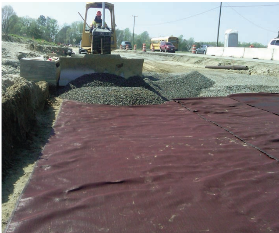
Placement of #57 stone over Mirafi® RS580i.
