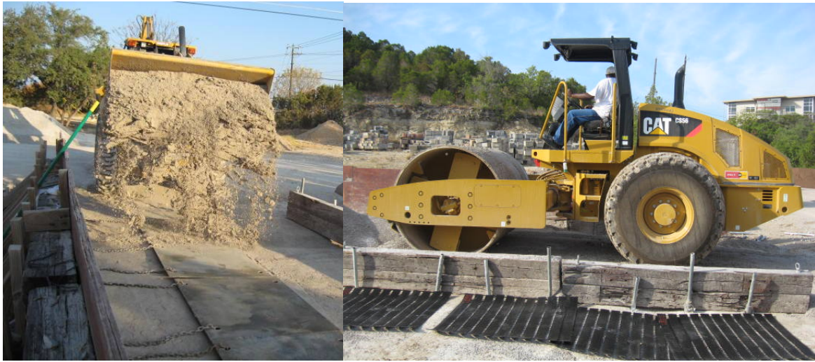
Figure D-1. Lifting Plates positioned between ties and covered with first lift of compacted soil/aggregate.
