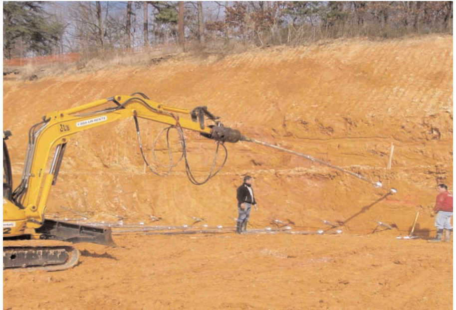
ABOVE: Anchor drilling into the side of the cut slope.
