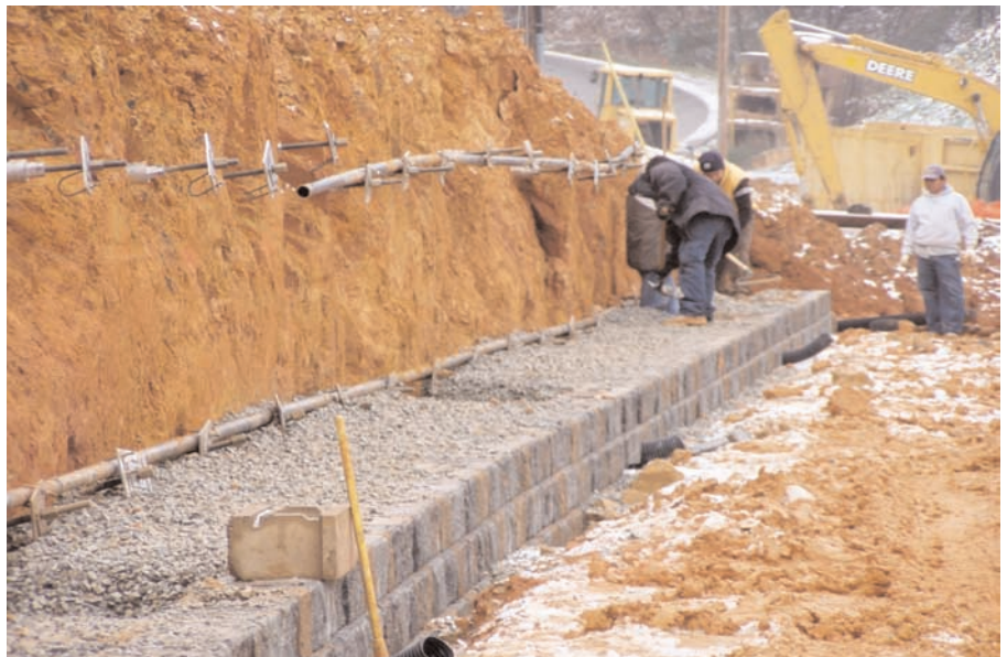
BELOW: Galvanized header-pipe being attached to the anchors.
