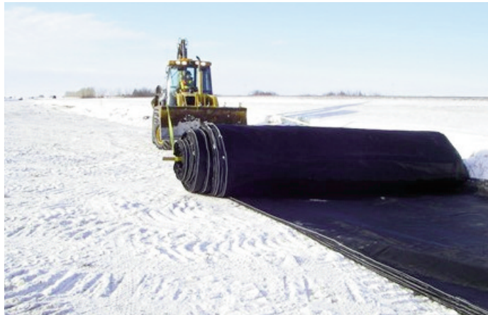
Figure 3 - Seaming panels being deployed over frozen slough surface
