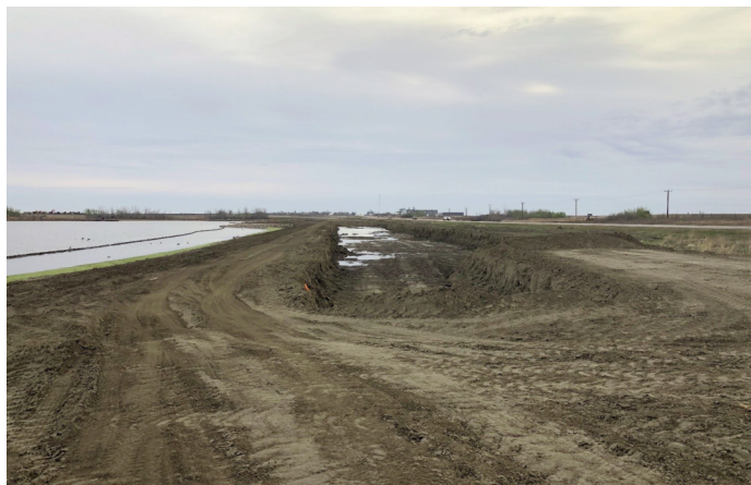
Figure 5 - Trenched embankment speeding up thawing of underlying ice
