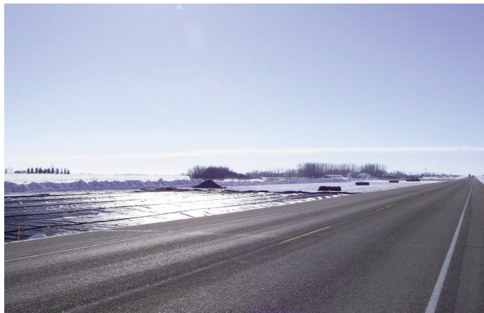
Figure 4 - Seaming panels being deployed over frozen slough surface
