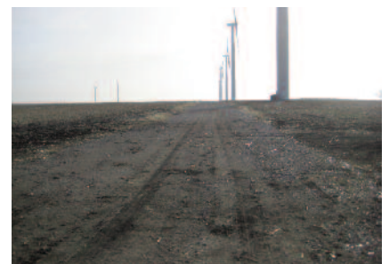
Road construction looking west using Mirafi® HP570 and 8" to 10" of limestone after 5 years.
