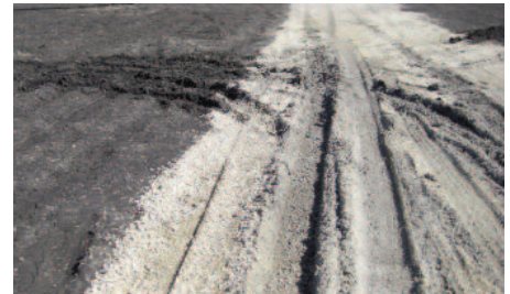
Break down of soil cement after 6 months due to freeze-thaw cycle and moisture.
