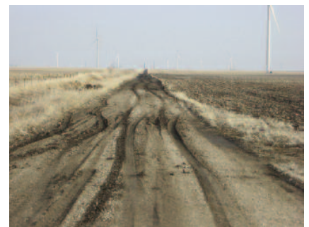
Road construction looking north using soil cement and 4" of limestone after 5 years.
