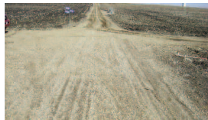
Road where soil cement and geotextile were used. Construction was completed and reviewed after 6 months. Note stone loss and rutting.
