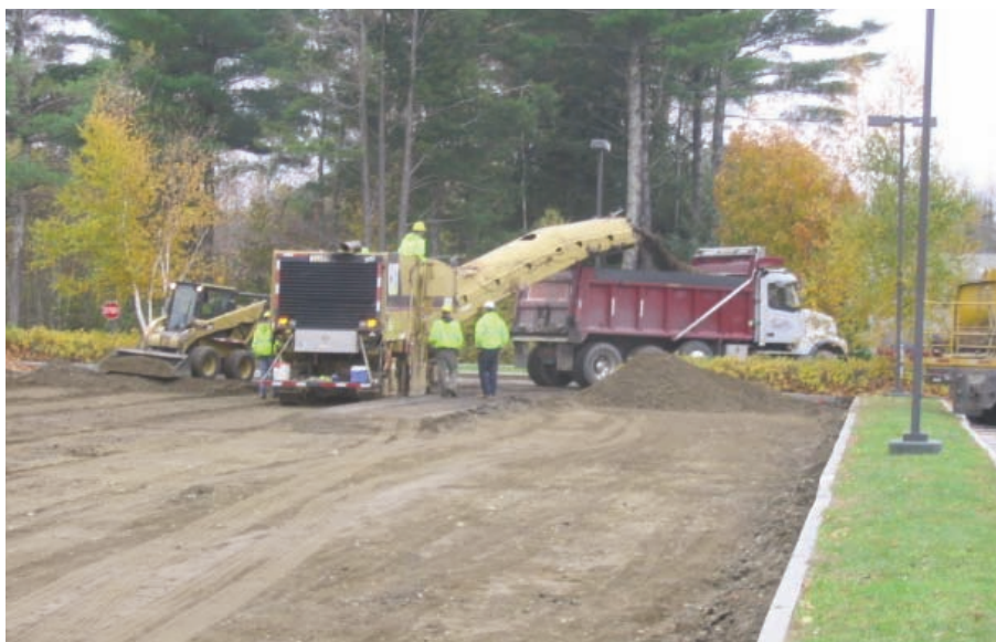
Recycling asphalt wearing surface.
