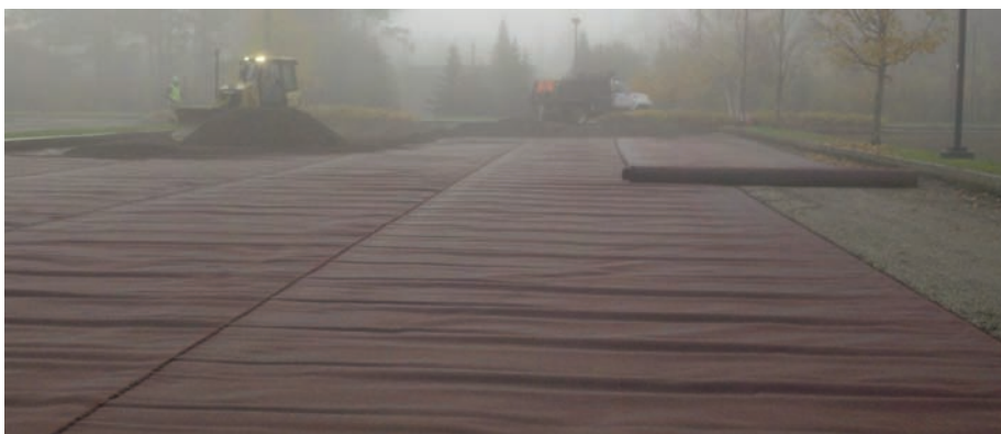
Installation of Mirafi® RS580i on soft soils in the parking area.
