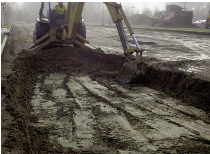
Preparation of subgrade for Mirafi® RS580i placement.
