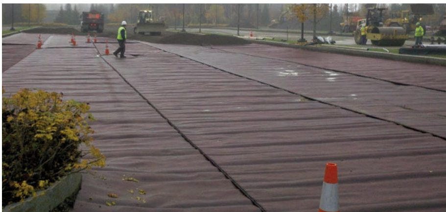
Installation of Mirafi® RS580i on soft soils in the parking area.
