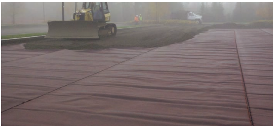
Base material being end dumped and spread on Mirafi® RS580i.
