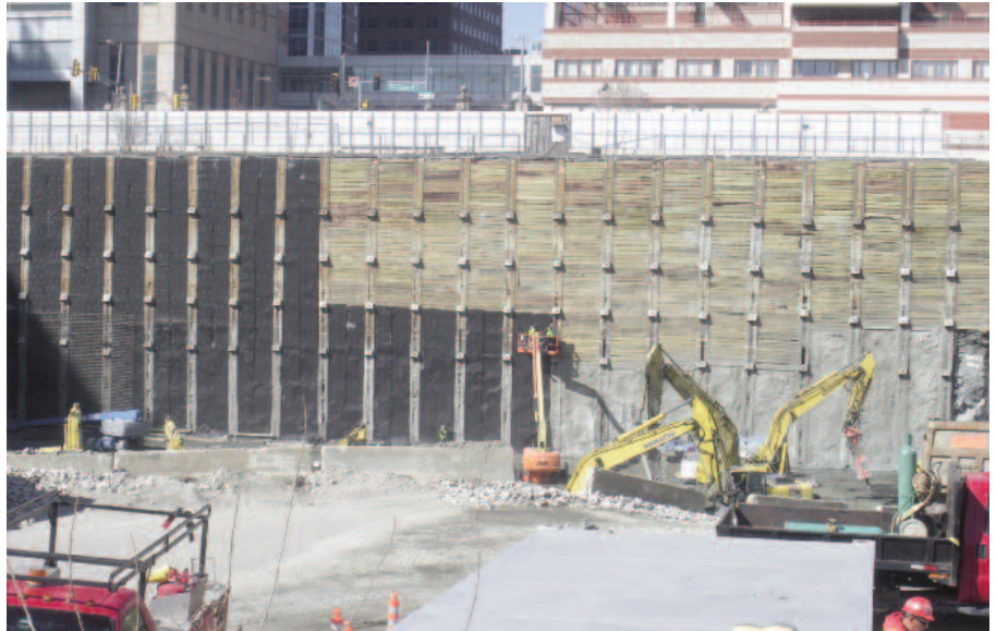
Placing Mirafi® G-Series drainage composite against lagging.
