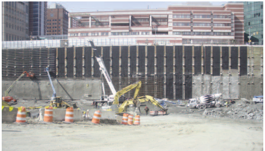
Placing shotcrete.
