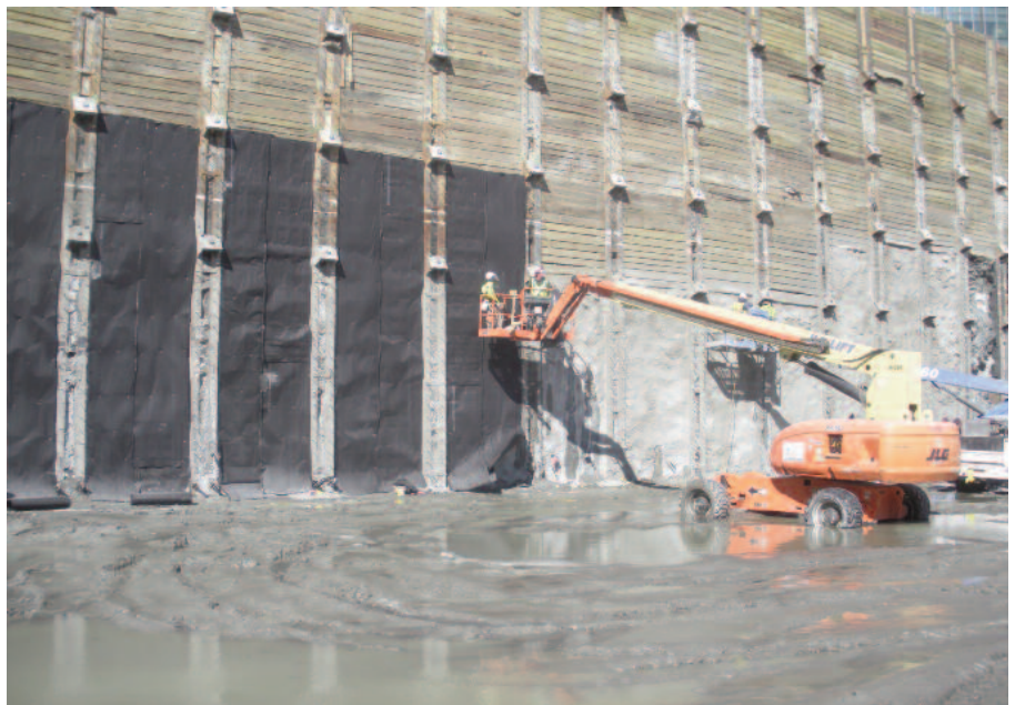
Mirafi® G200N placed over shotcrete.
