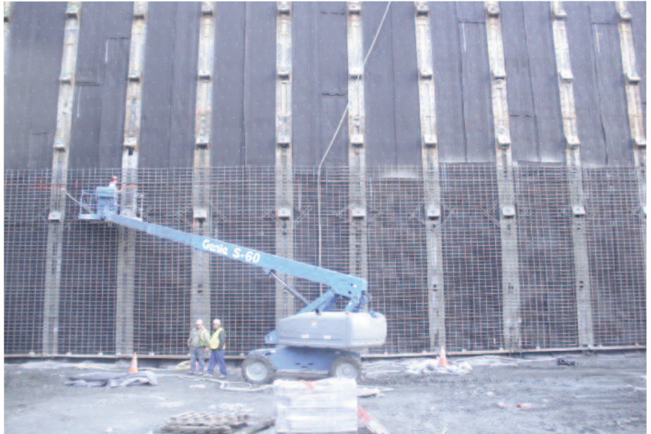
Placement of rebar mat to receive shotcrete.
