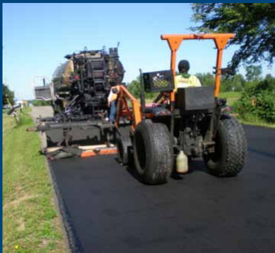
INSTALL FABRIC OVER LIQUID ASPHALT
