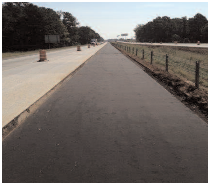
Roadbed covered with Mirafi® 1450BB ready for cement paving.
