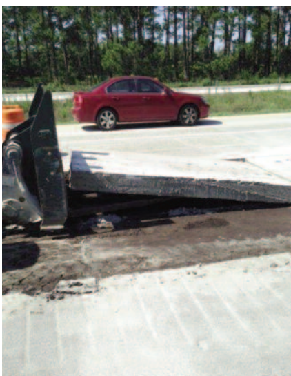
Removal of the existing concrete roadway.
