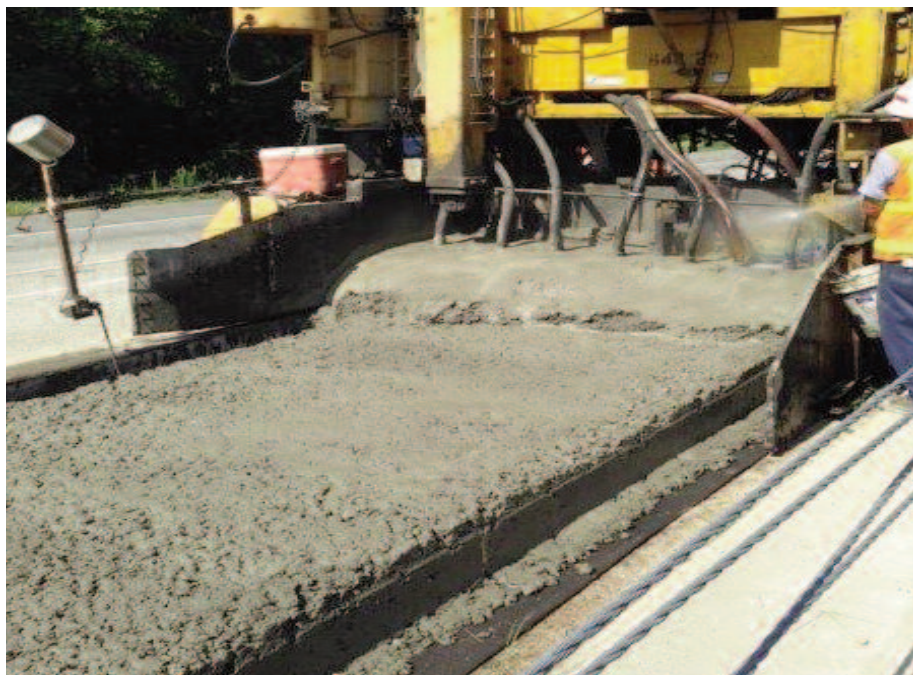
Paving of new wider cement shoulder over Mirafi® 1450BB.
