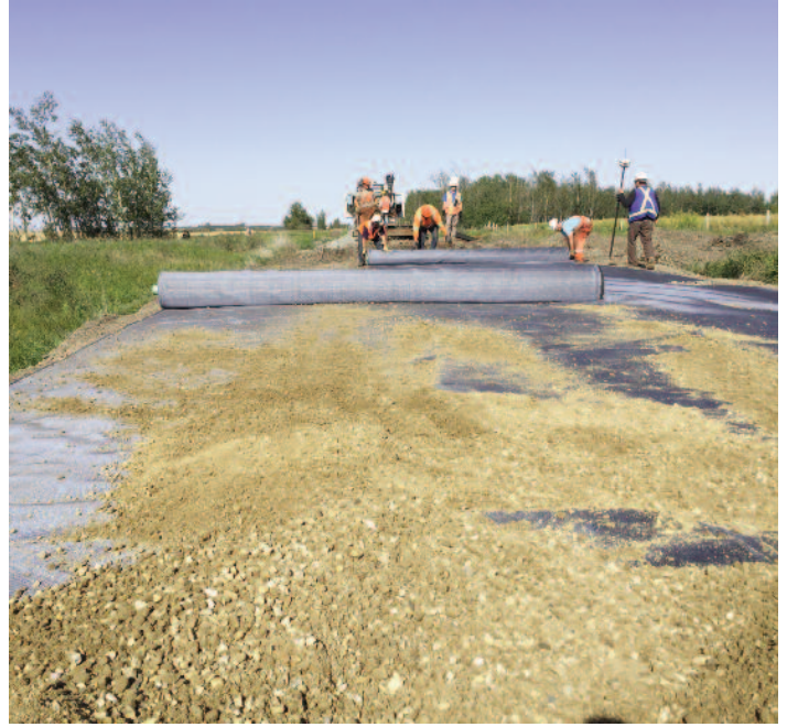
Mirafi® H2Ri installed at the subgrade/subballast interface.
