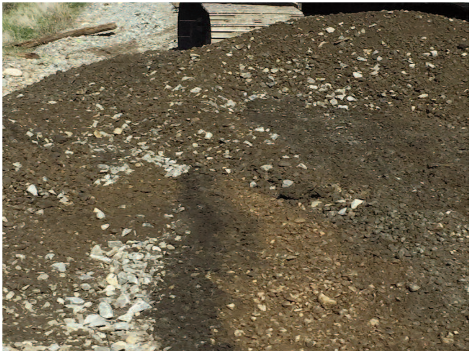
Contaminated rail ballast: The dark material is topsoil that has migrated into ballast. The lighter area is sub-ballast, which has migrated into ballast.
