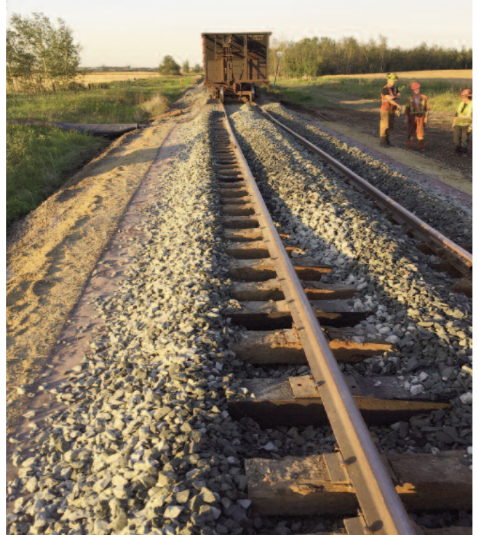
Placing new ballast.
