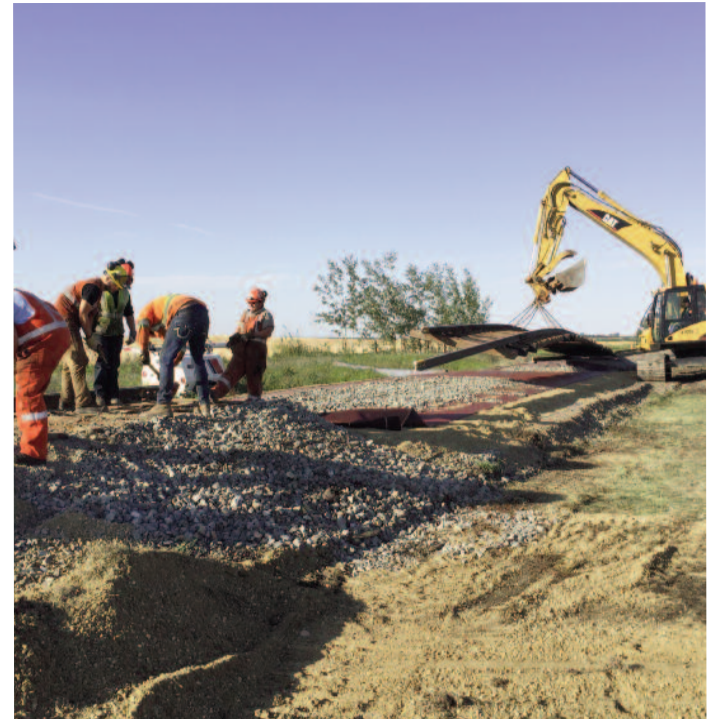
Reconnecting the track panel.
