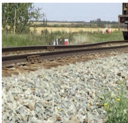
Unrepaired track section with cross level variation due to settlement issues.
