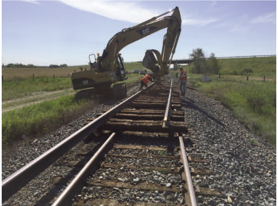
Track panel is removed.
