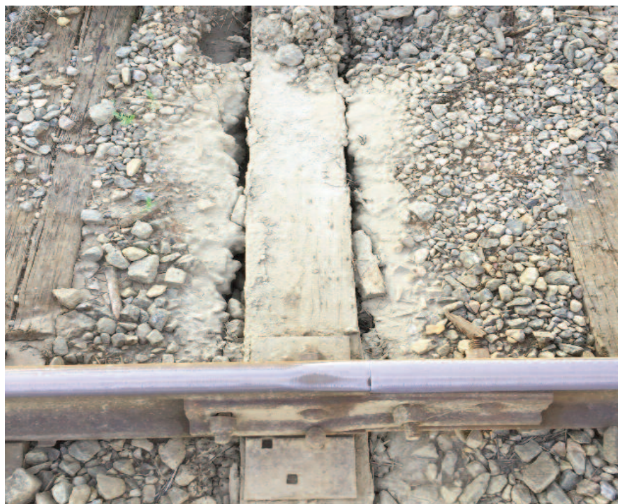
Evidence of mud pumping and ballast contamination prior to repair.
