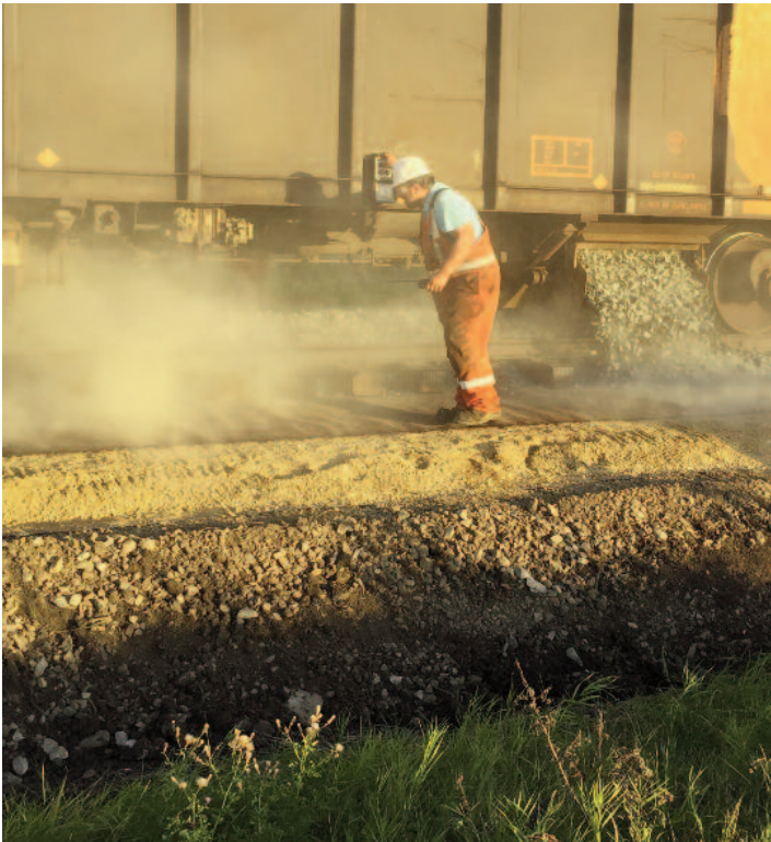
Placing new ballast.
