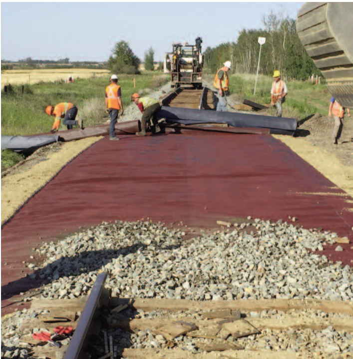
Mirafi® RS580i installed at the ballast/sub-ballast interface.
